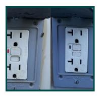
**ISSUE:** Due to extra electrical power demands in the winter, a GFCI may trip and no longer provide power to a heat trace line, pump heater or the pump itself.
