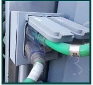
**ISSUE:** Sometimes our heat trace is unplugged from the outlet to make room for an engine block heater. Make sure all lines are plugged in.
